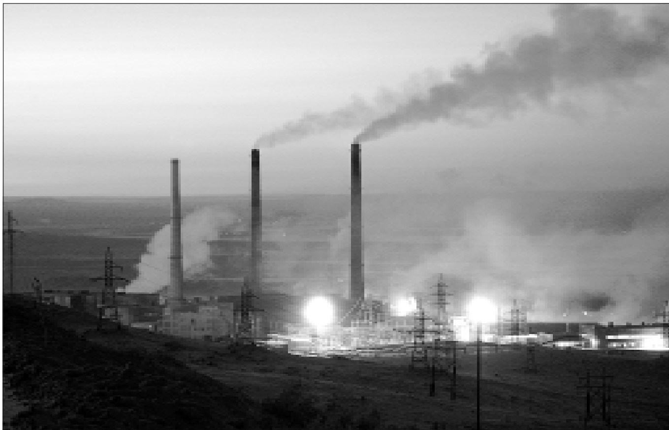
THE NIKEL SMELTER, NORWAY IN THE BACKGROUND, DECEMBER 2002. PHOTO BY RAGNAR VÅGA PEDERSEN, SVANHOVD MILJØSENTER, WWW.SVANHOVD.NO
