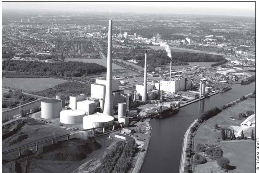
Fynsværket in Odense runs on coal, oil and natural gas. It has an output of 640 MW and produces electricity and district heating. The plant is equipped for flue gas desulphurization and emitted 970 tonnes of sulphur dioxide in 2004. With a specific emission level of 27 mg SO 2 /Nm 3 the plant was well below the 400 mg/Nm 3 limit value.
