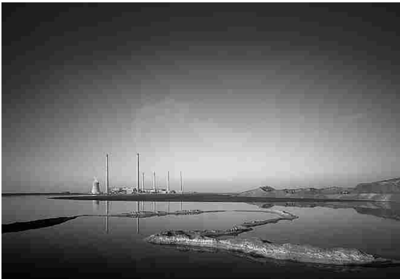
MARITSA POWER PLANT, BULGARIA. © MICHAEL REINHARD
