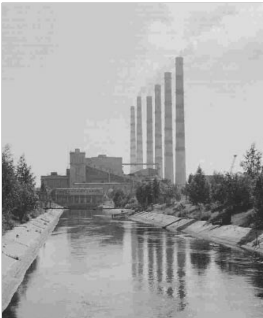
BALTI POWER PLANT. PHOTO BY EESTI ENERGIJA
